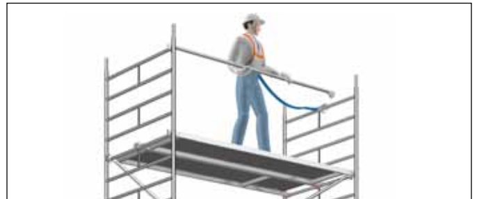
Fig. 3: Safe assembly of rear guardrails using PSA
