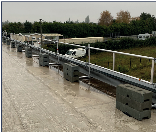
Compact flat roof edge protection assembled with rolling tower guardrails.
